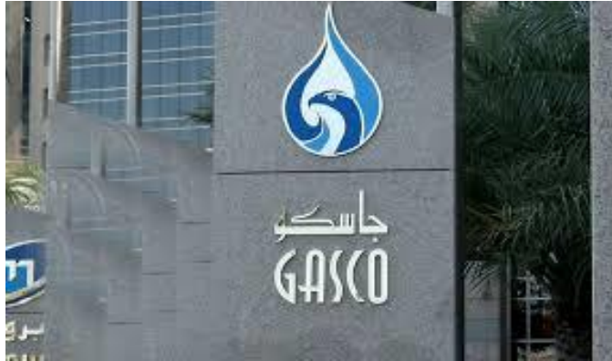
GASCO (ADMINISTRATION BUILDING DAMIETTA).
