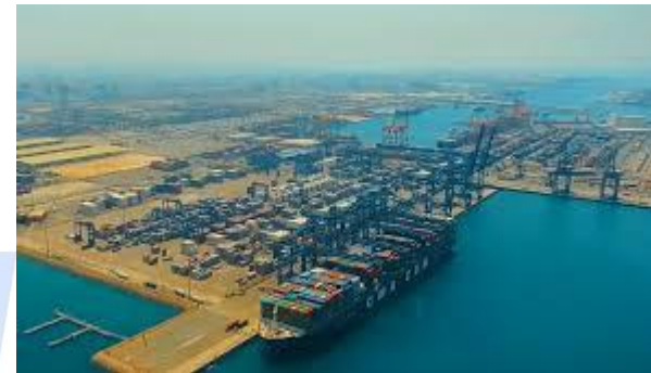
SAVOLA QUENCH IN JEDDAH ISLAMIC PORT, JEDDAH, SAUDI ARABIA
