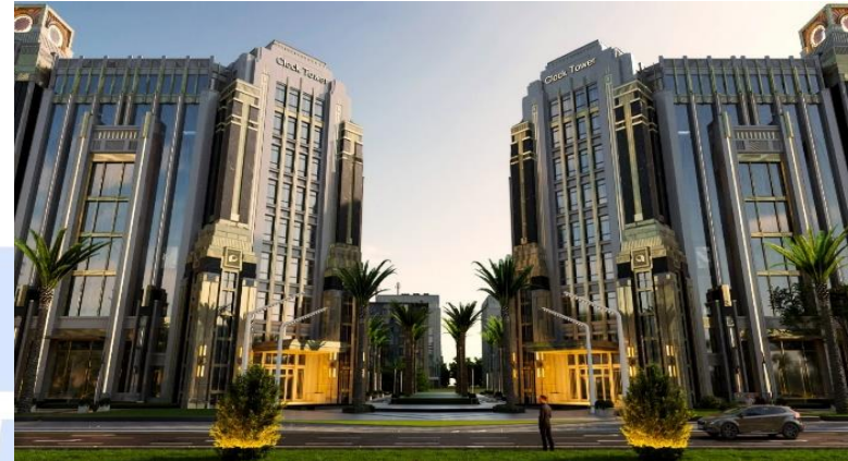
CLOCK 3 TOWER ADMINISTRATION BUILDING
