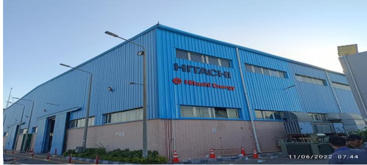
HITACHI TRANSFORMERS FACTORY, 10TH OF RAMADAN. EGYPT
